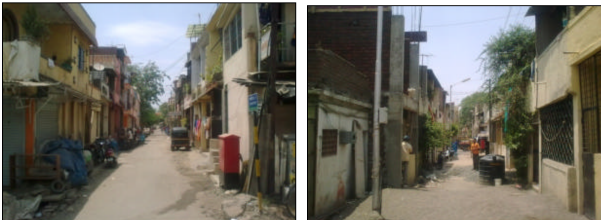
Figure 6.30: Showing current development of Bibwewadi housing
