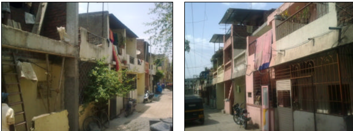
Figure 6.29: Showing current development of Bibwewadi housing
