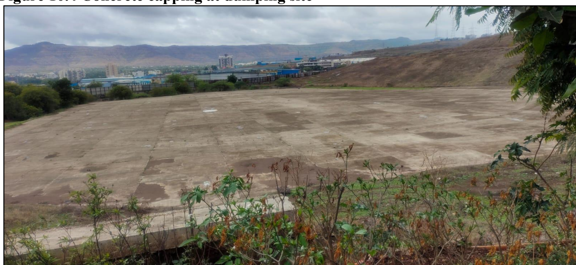
Figure 10.4 Concrete capping at dumping site
