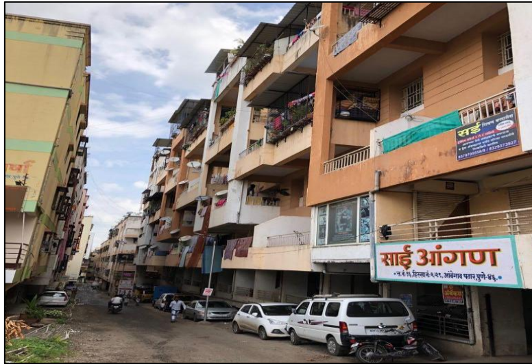
Figure 4.34 Dense development - Ambegaon Budruk
