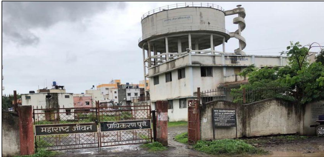
Figure 4.13 Water treatment plant located at Shivane-Uttamnagar
