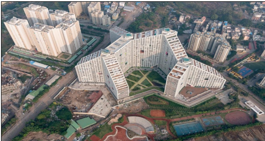
Figure 4.15 Recreational Facilities - Amanora Township, Hadapsar
