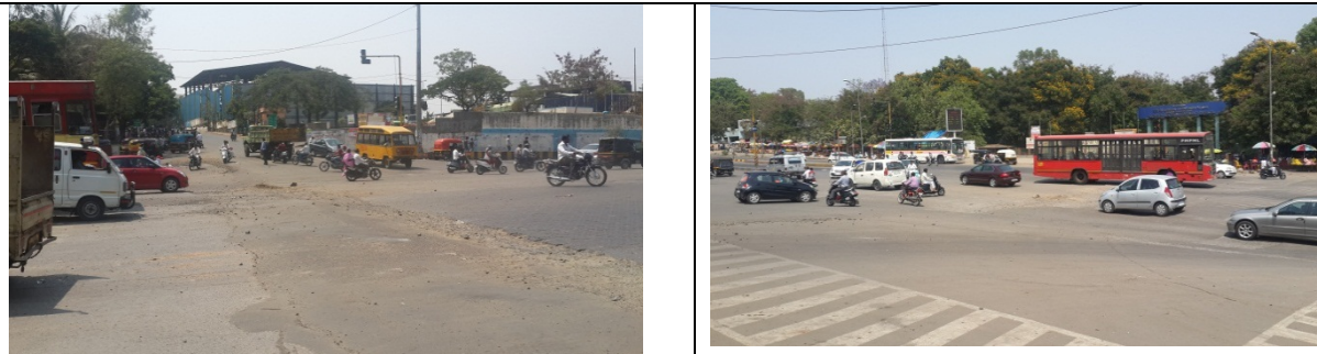
Katraj Zoo junction (Chainage 0/800 m 18.454435, 73.858613)– Cross cut taken by MNGL has left the main carriageway in poor condition and unattended. Driving conditions are extremely hazardous. There is lack of channelization at this wide junction creating chaotic situation. There is no provision for a pedestrian crossing in this stretch where the road is 60 m wide at the junction.
