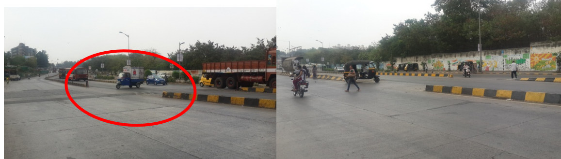
Chainage 0/400 m LHS side – Break in the BRTS corridor at minor cross road gives access to all other vehicles to cross the BRTS corridor creating unsafe driving condition for the BRTS buses as well as the other vehicles.
