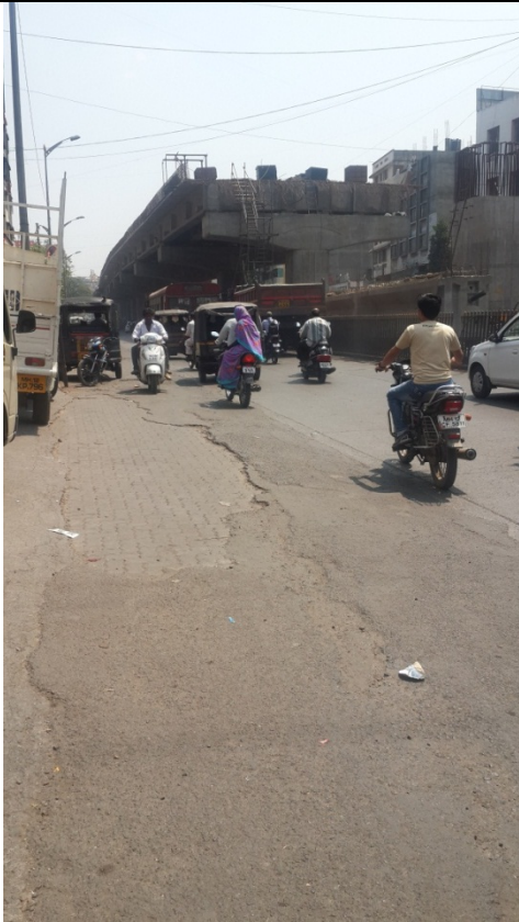
Construction zone Dhankawadi flyover (Chainage 2/350 RHS side 18.465086, 73.858158)– The edge strip of 3 to 3.5 m (one lane) is in a bad condition and needs to be replaced / repaired by eliminating the level difference which tends to lower the speeds of two wheelers and other vehicles and results in congestion. Parking in this area needs to be banned until the completion of flyover.
