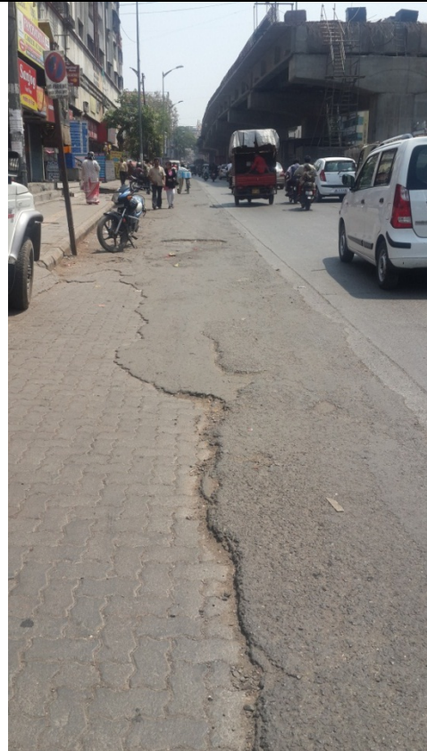
Construction zone Dhankawadi flyover (Chainage 2/350 RHS side 18.465086, 73.858158)– The edge strip of 3 to 3.5 m (one lane) is in a bad condition and needs to be replaced / repaired by eliminating the level difference which tends to lower the speeds of two wheelers and other vehicles and results in congestion. Parking in this area needs to be banned until the completion of flyover.
