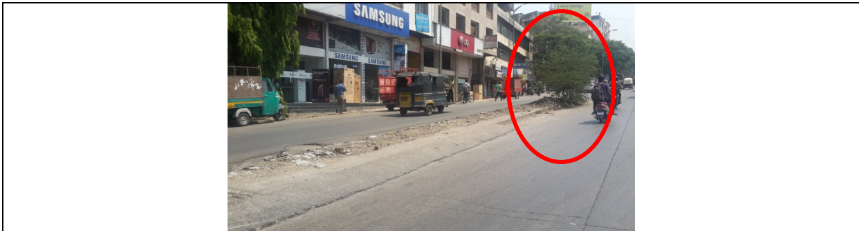
Chainage 1/650 RHS side 18.460663, 73.858184: A tree in between the main carriageway and service road obstructs vision and poses danger to oncoming traffic.
