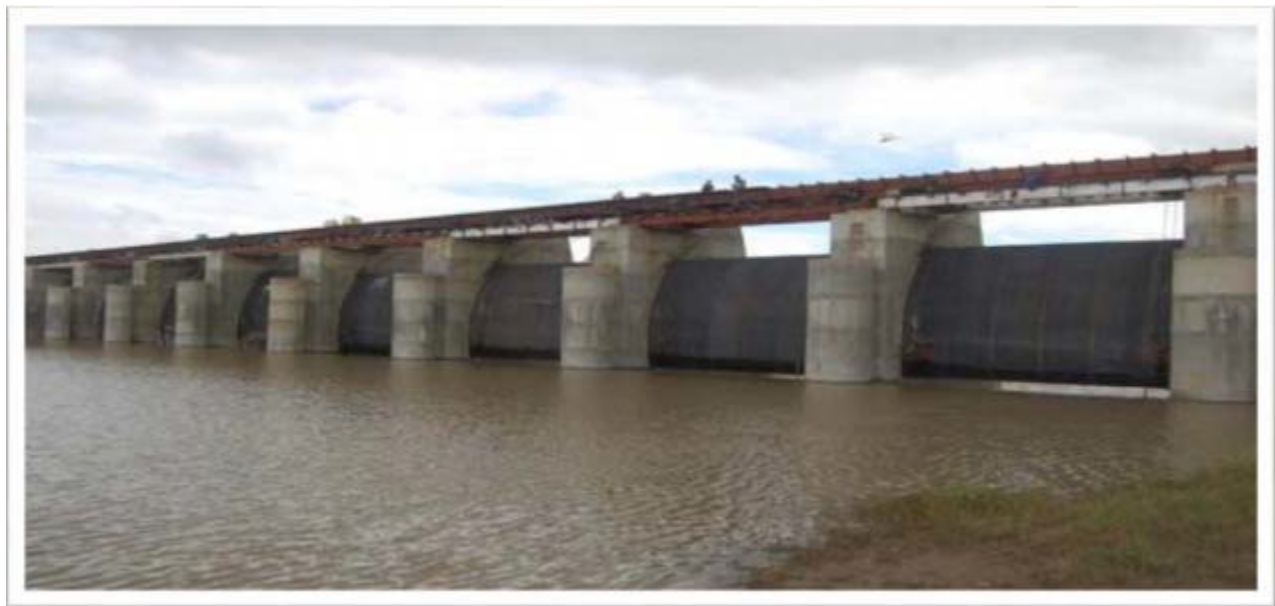
Figure 35 : Typical Barrage Photograph
