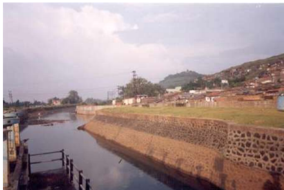
RIGHT BANK CANAL AT PARVATI
